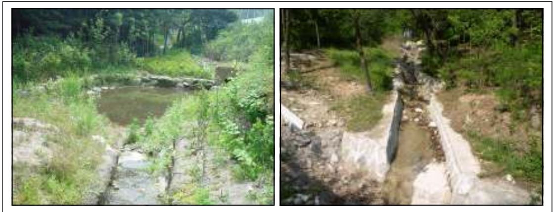
Fig. 14. Example for at the valley check dam construction(Mt. Nam).
